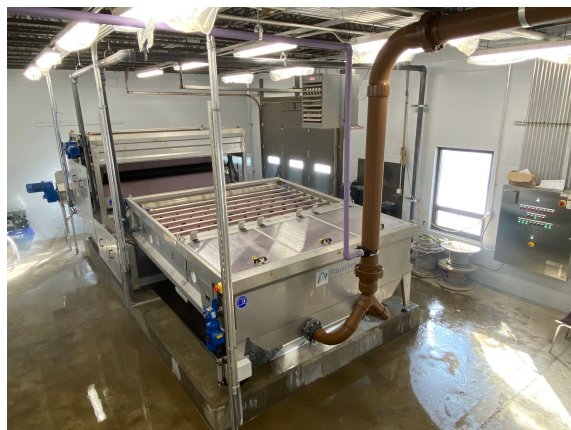
Omega NHP in a municipal dewatering building
