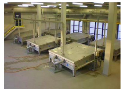
6 sets Gravity Belt Thickener OMEGA 30 MD
